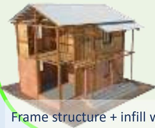
Frame structure + infill wall
