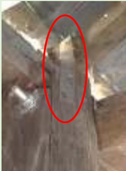
Note : 3 mm thick metal strap, Minimum four numbers of 50 mm long nails (Fe250) with Floor member and Minimum four numbers of M16 grade expansion bolts with walling material
